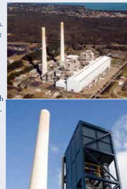
Munmorah Power Station, and below the Post combustion capture (PCC) pilot plant built by Delta Electricity and CSIRO. image: air shot by Delta Electricity; image of pilot below by CSIRO
