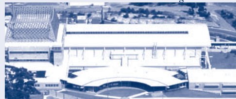
The new OPAL reactor building
