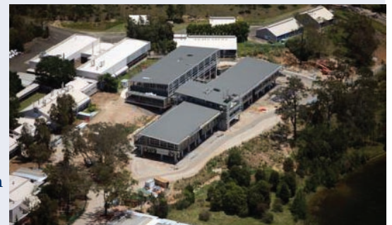
Aerial photo of the Elizabeth Macarthur Agricultural Institute, Camden, Sydney – the only high containment animal, plant and aquatic bio-security diagnostic facility in NSW. image: NSW Public Works
